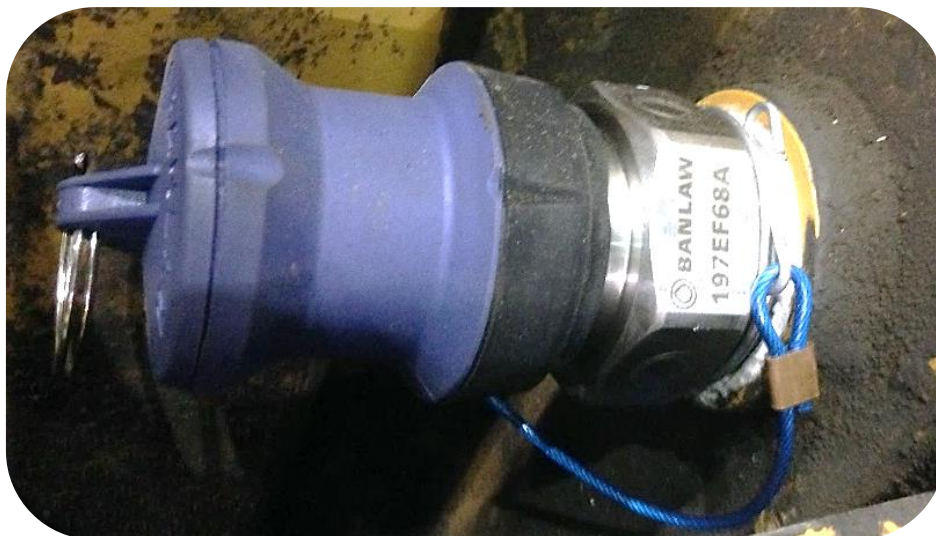
Figure 16 - Banlaw Receiver Installed with Dust Cap
