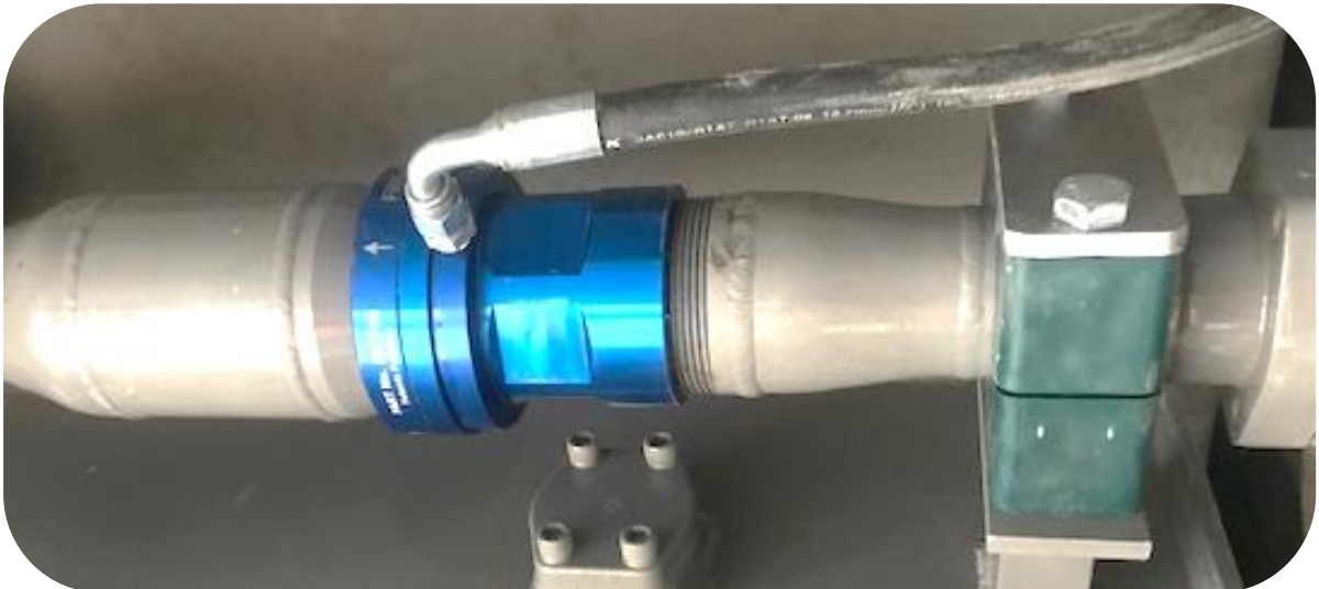
Figure 15 - Example of BFCV80 Installed
